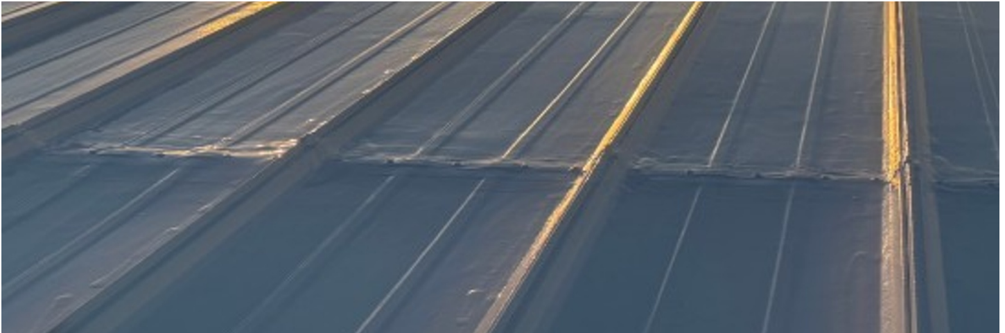
Restored R-panel metal roof
