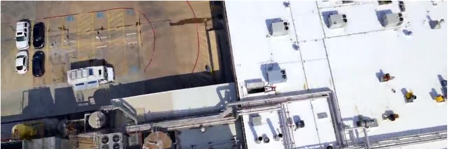
Completed roof restoration
