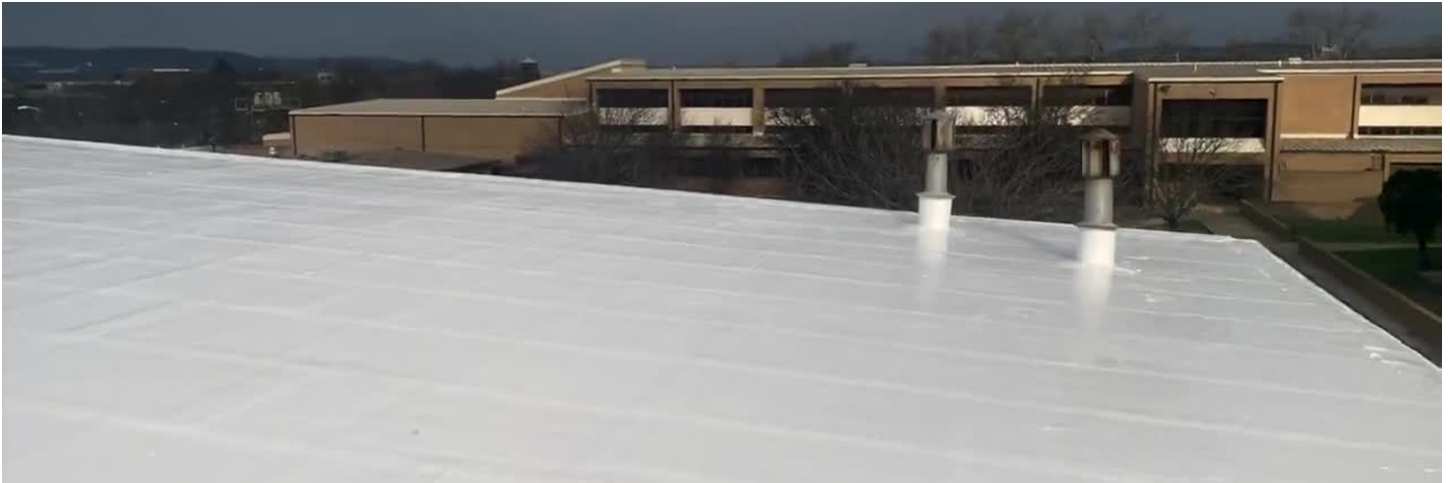
Completed roof restoration
